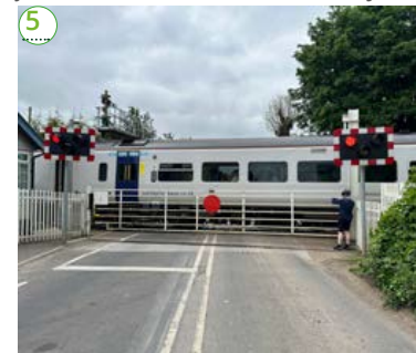
5 Cattal Station Crossing
